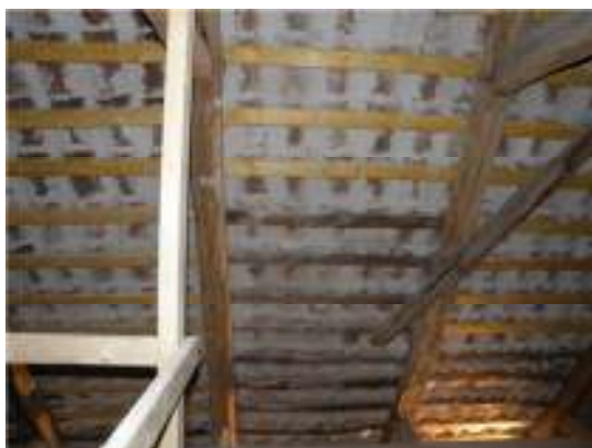
Norra takfallet understruket.
